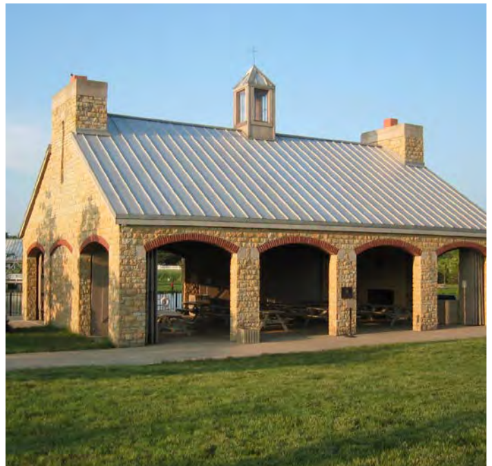
Covered structures can offer informal spaces for social gatherings gatherings and events, or even warm weather concessions and rentals.
