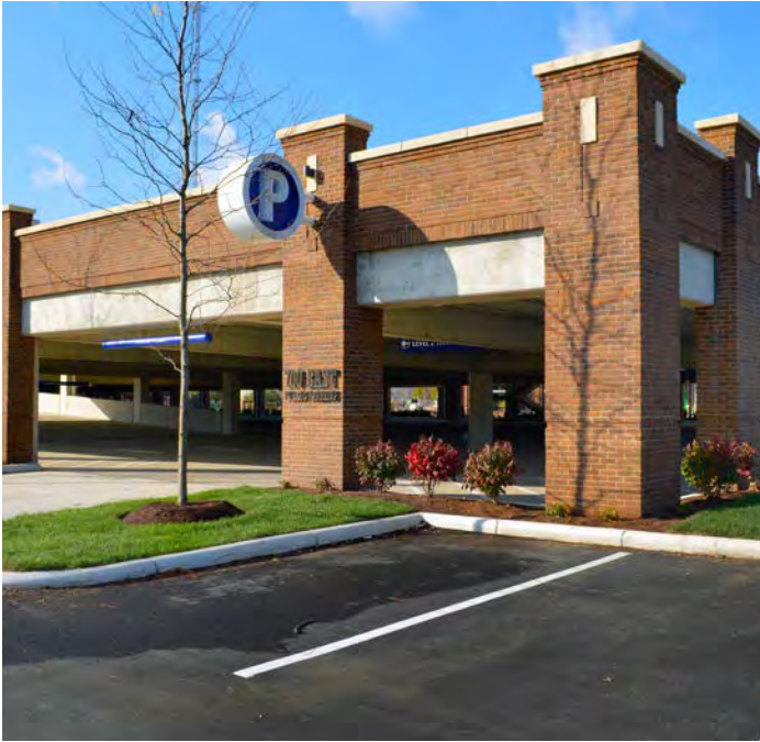
Parking decks offer an affordable way to double surface parking yields while avoiding the creation of new surface parking lots.
