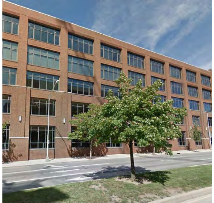
Example of parking garage that provides street-level detailing and interest, including windows and architectural lighting. The first floor can be active storefront uses.
